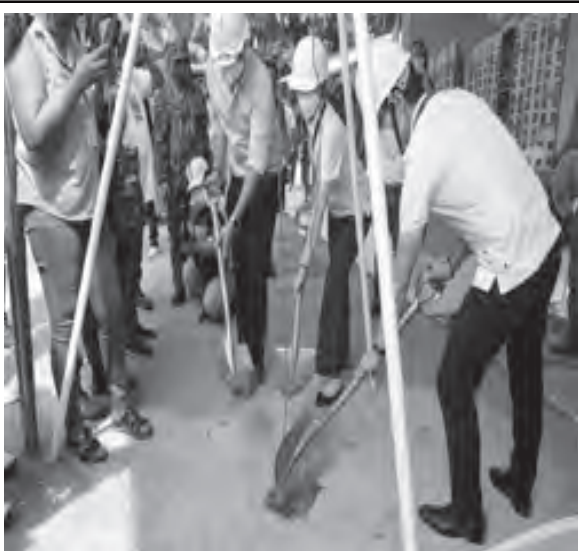
PINANGUNAHAN nina Manila City Mayor Fransisco ISKO Moreno Domagoso, Bise Alkalde Honey Lacuna Pangan, at City Engr. Armando Andres ang Ground Breaking Ceremony ng itatayong TONDINUIM 1-2 na tatawaging Vitas City Vertical Housing na may taas na 15 palapag, 44 sq meters laki at 336 units para sa mamamayan ng Tondo, Maynila. (Christian Heramis)
