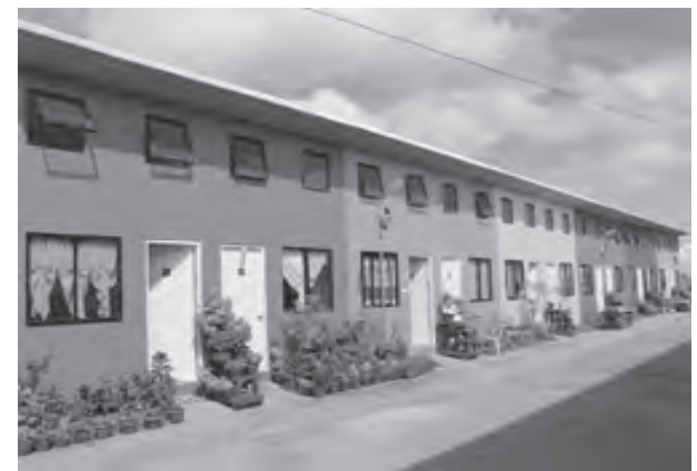
The SM Cares Village in Bogo City, the first of the four Villages constructed by the SM Group, is located in a one-hectare lot in Barangay Polambato, Bogo City.
